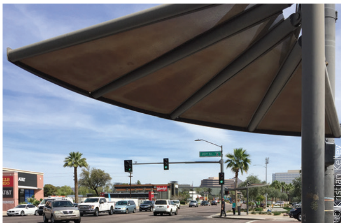
Figure 3 Perforated screen parallel with roadway provides shade on one side at all times of day. The perforation is necessary to allow views into the shaded space for security. Photo Source: Kristian Kelley
