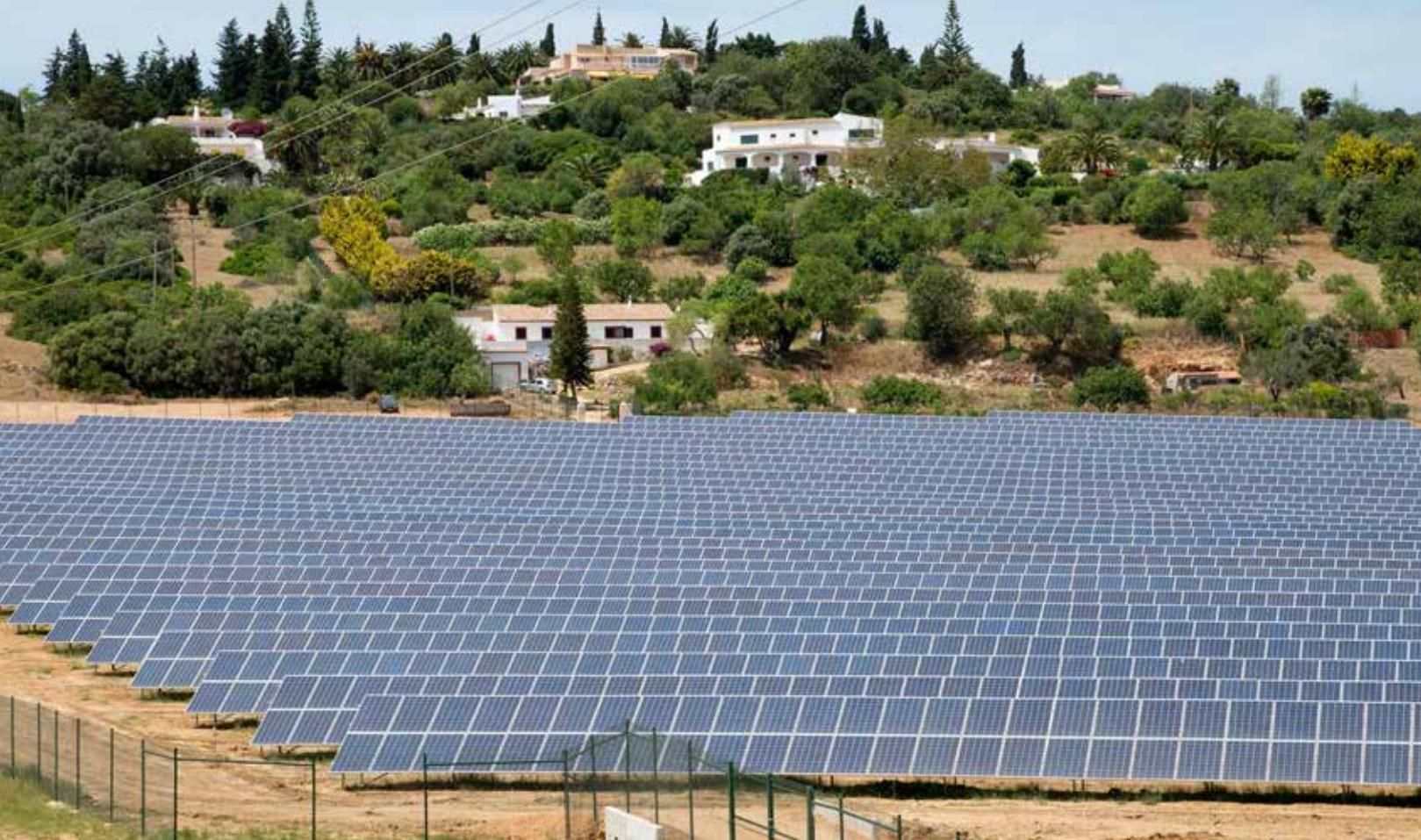
© PETE TITMUS/ALAMY STOCK PHOTO (COMMERCIAL SOLAR PANELS, PORTUGAL)
